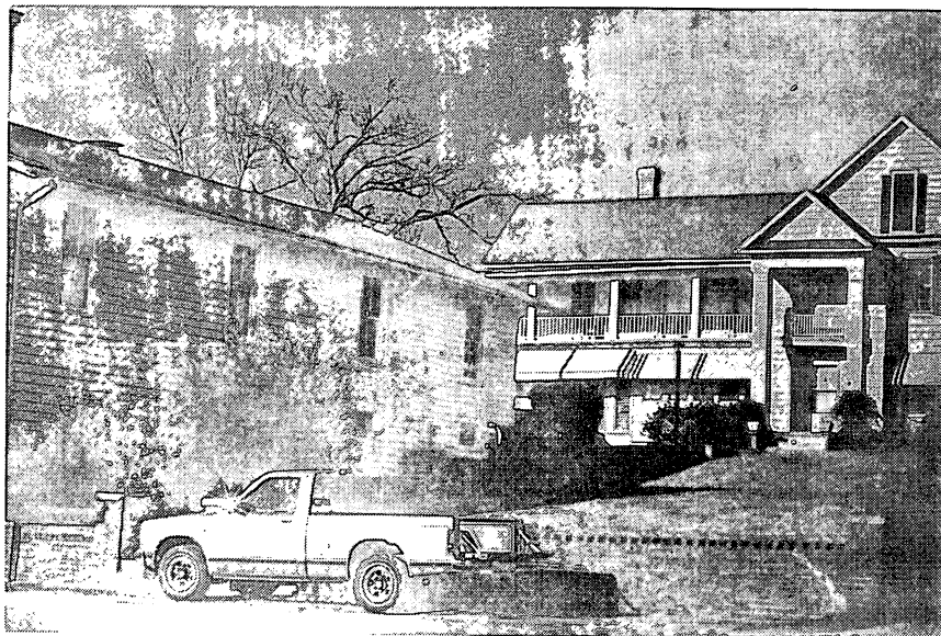
Plate 4. Pelletier House, Looking North.
